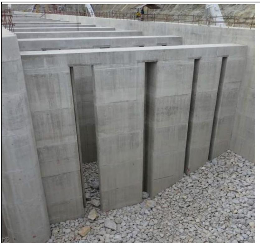
*Figure 1: Vertical slot component of upstream fish pass (Source: Coe 2015 Xayaburi HPP: Fish Migration Facilities”, Pöyry and Fishtek [V1])*
