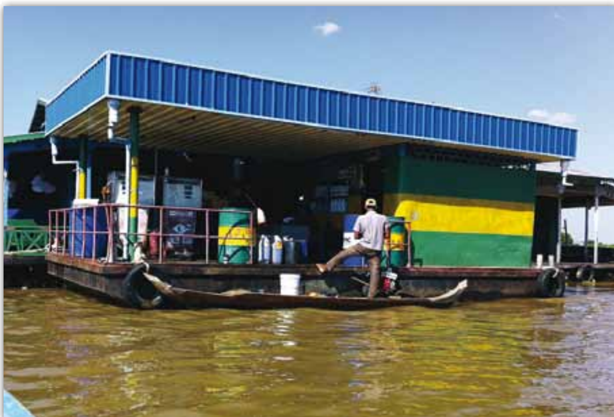
Figure 39: Floating Fuel Terminals on Tonle Sap Lake, Cambodia
