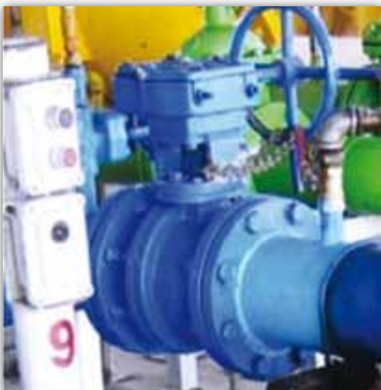
Figure 19: Manually-Operated Valves
