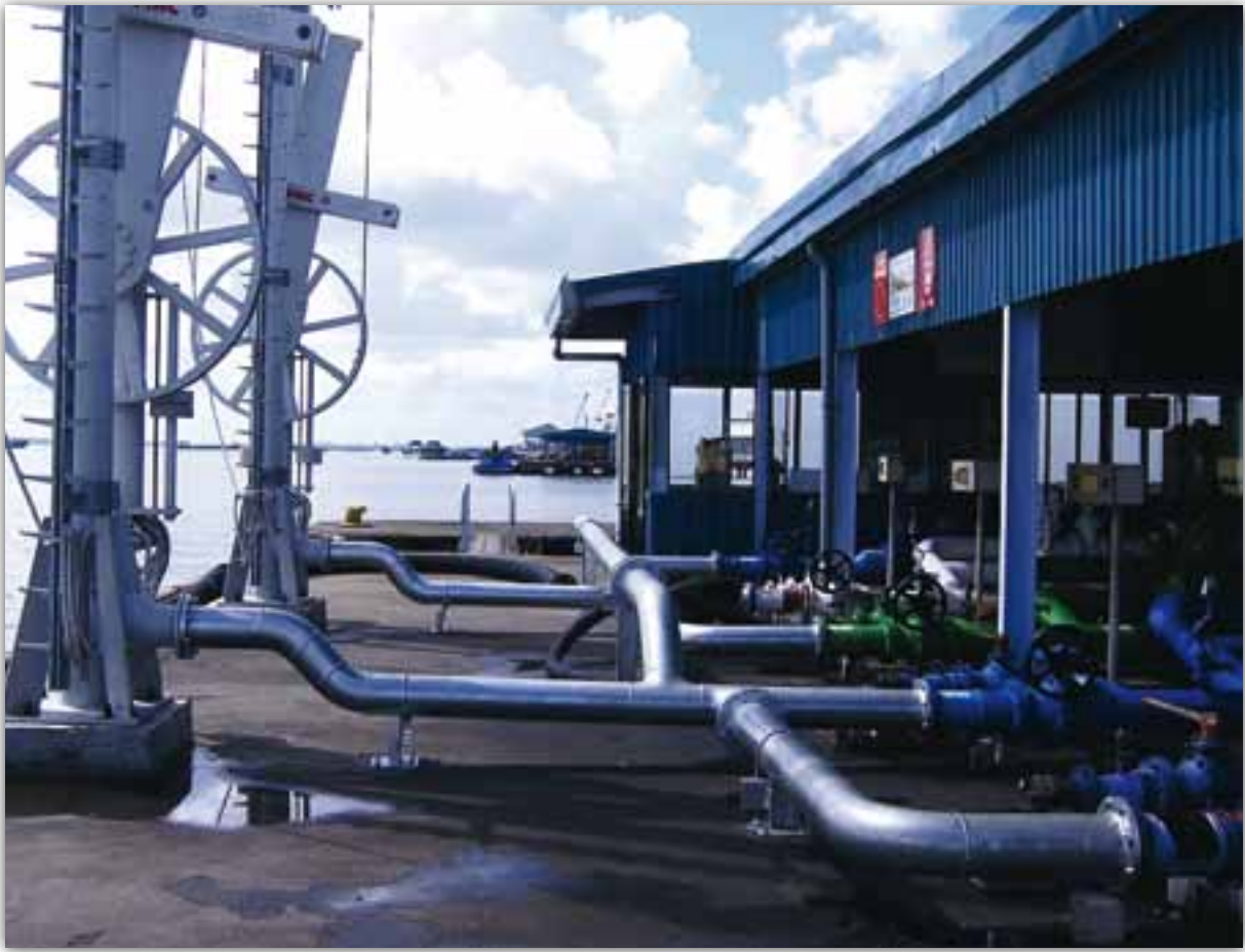
Figure 59: Example of Cargo Pipes at a Typical Vietnamese Terminal
