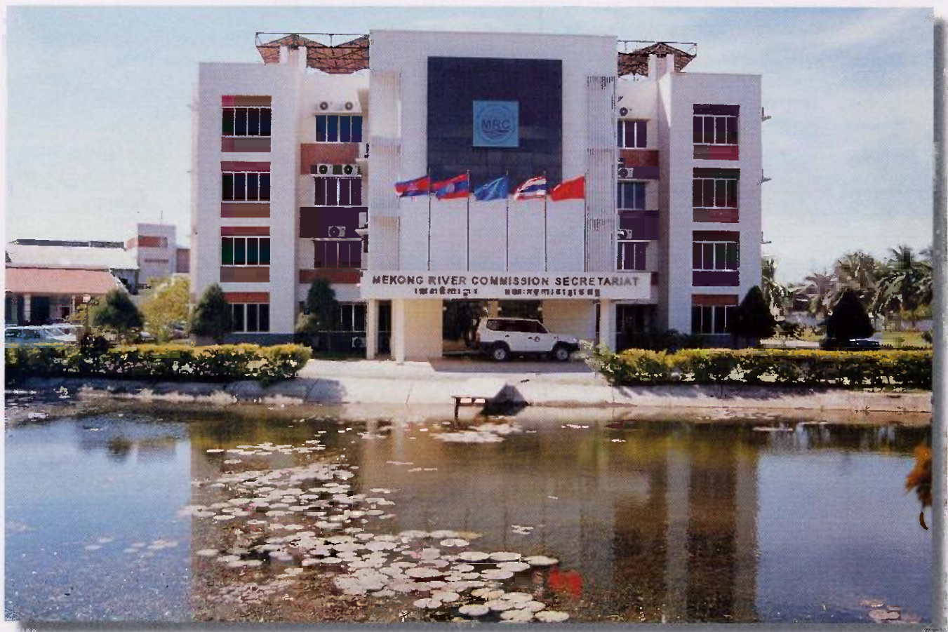
New Headquarters of the Mekong River Commission, Phnom Penh
