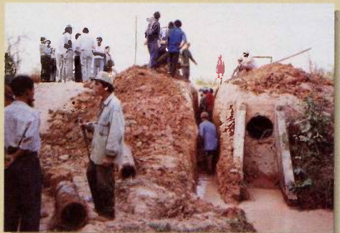
Improving canal system at Nakung-Thunlua Pumping Scheme, the Lao PDR.
