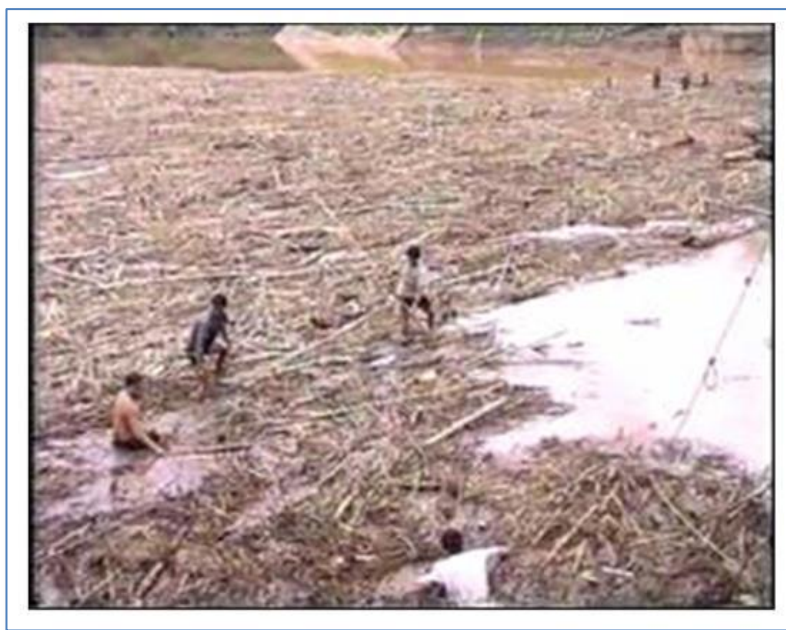
Figure 2-3 An indication of the debris loads carried by flash floods. Trash being cleared after being trapped in Luangnamtha diversion weir, Lao PDR, during an event in 2006.
