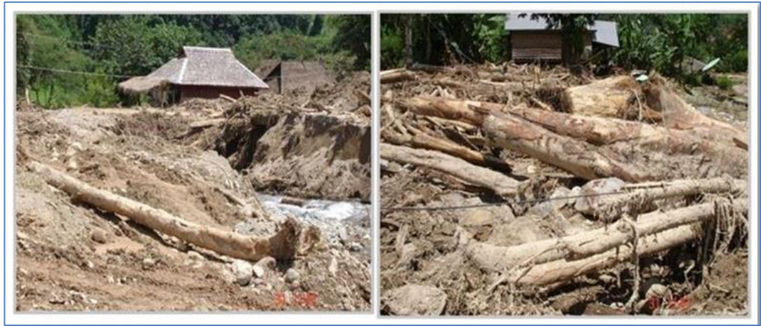
Figure 2-5 Channel blockages caused by a flash flood in the Long District of Luangnamtha Province, Lao PDR, last week of August, 2010.
