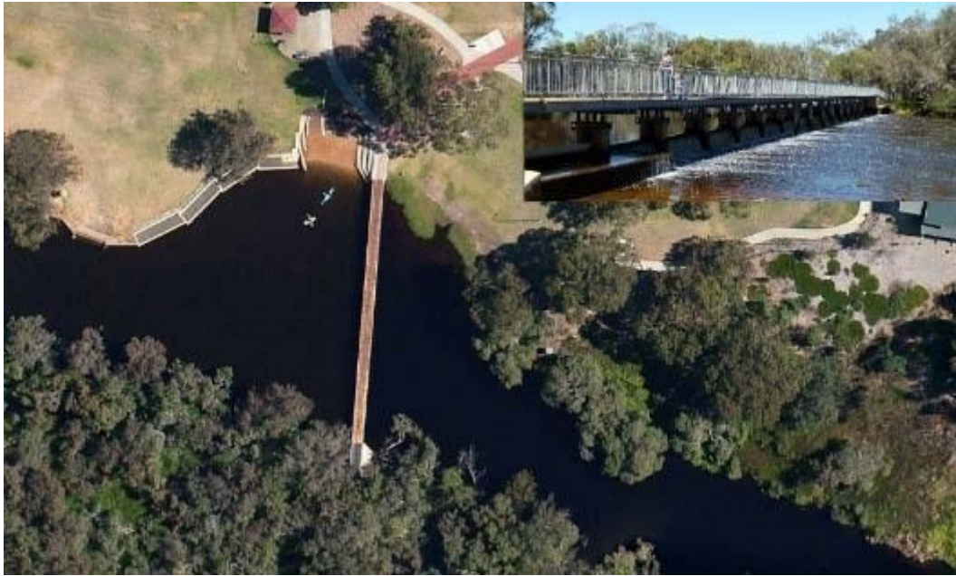
Figure 37. A weir hidden beneath a bridge.
