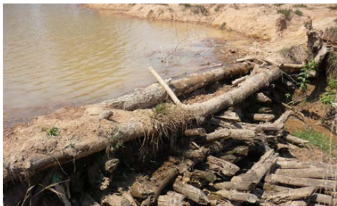
Figure 40: Earth weir in Lao PDR
