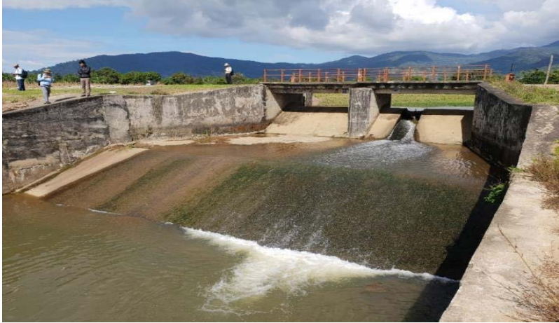
Figure 46: Low flow at a weir at the end of the wet season
