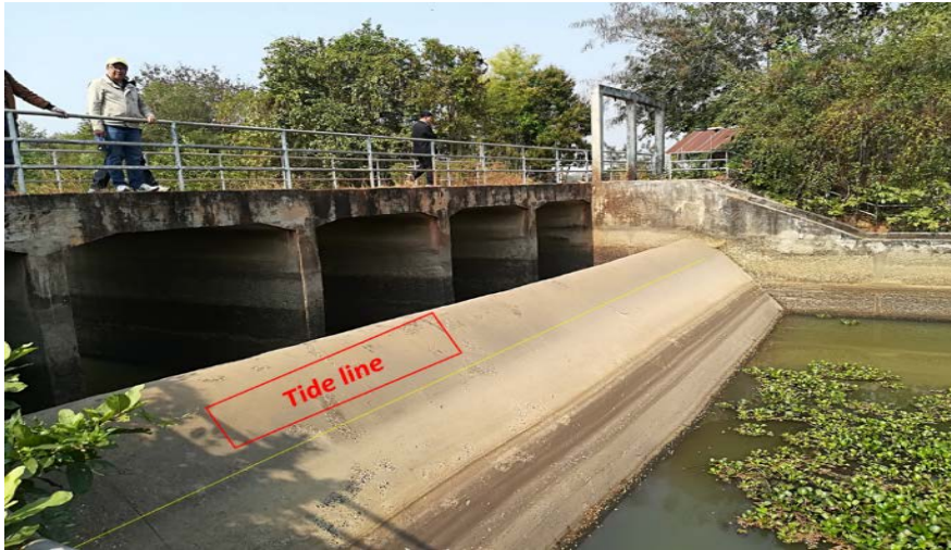
Figure 44: Tide line of a weir
