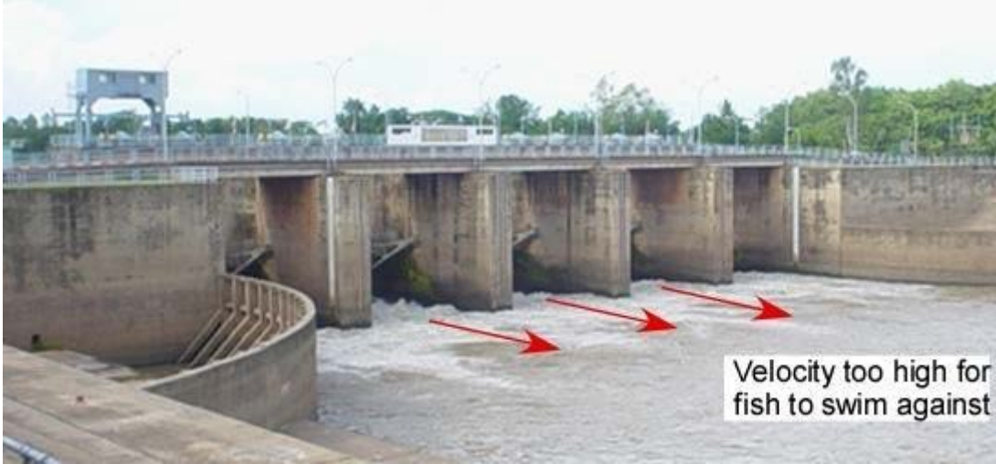
Figure 30. Radial Gated Weir located on a major river has high velocity that fish cannot swim against.
