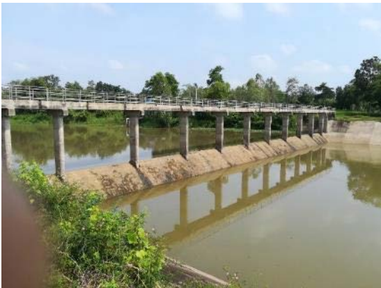
Figure 42 :Yes- The weir blocks fish migration. Figure 43: No- The bridge does not block fish migration.
