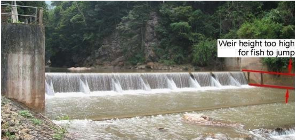
Figure 28. Typical run of the river weir located on an upland stream that is too high for fish to ascend.
