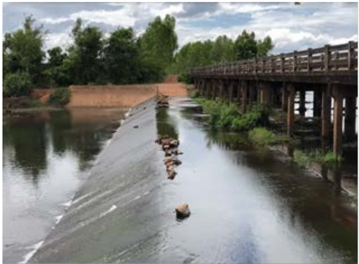
Figure 36: Bridge with a fixed crest
