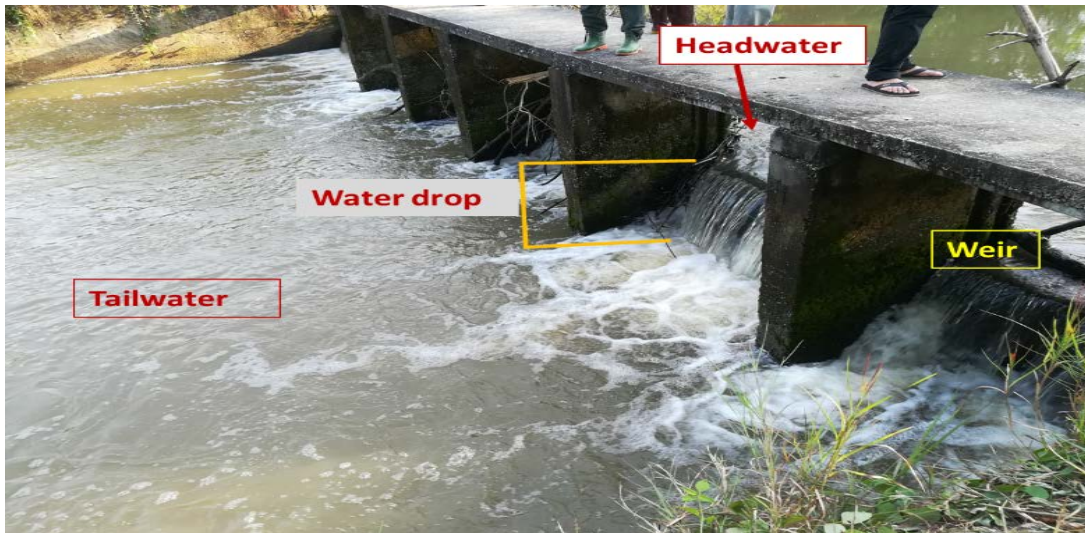
Figure 45: Tailwater, headwater and water drop of a weir which impacts upstream migrating fish
