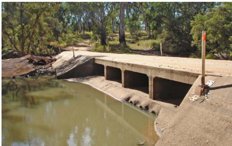
Figure 38: Culvert with shallow water flow and high drop
