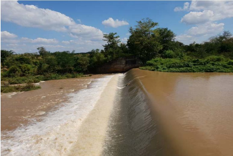
Figure 47: High flow at a weir in the wet season
